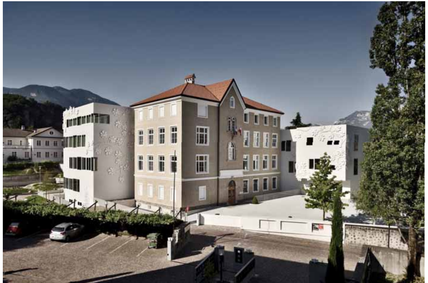
Elementary School, Renovation and Addition
